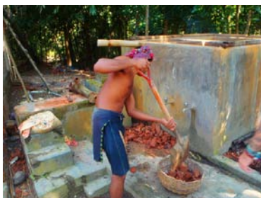
A local volunteer refurbishing a water filter
